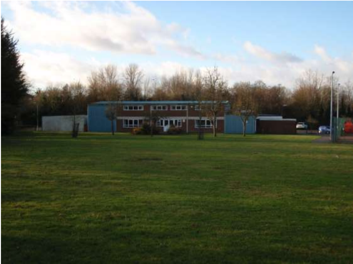
Plate 11. View to the south-west from the rear of the community centre
